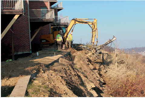
8 2012 年普赖斯山某区域的修复工作，该区域在邻近盆地西边公寓的位置发生严重塌方 Remediation work on a hillside in 2012 that collapsed perilously close to condominiums west of the basin in Price Hill
