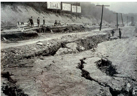
5 哥伦比亚林荫大道工程所导致的 1930 年滑坡 Landslide in 1930 resulting from development of Columbia Parkway
